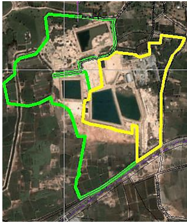
Surface Facilities Area for Camallite Processing
